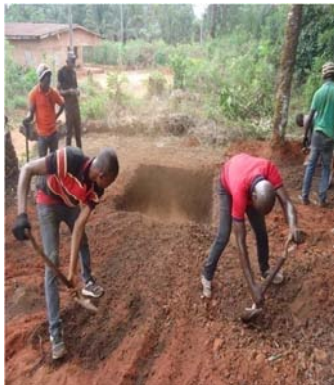
Figure 25. Covering of the trench.
