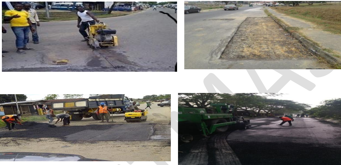
Fig.3 Cutting and patching of affected road pavement
