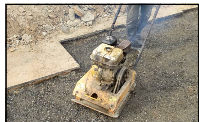
Fig. 17: Stone base was put, wetted and compacted.
