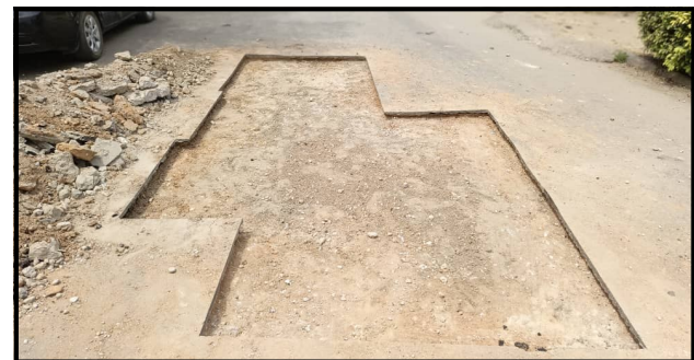
Fig. 15: The finished excavation.
