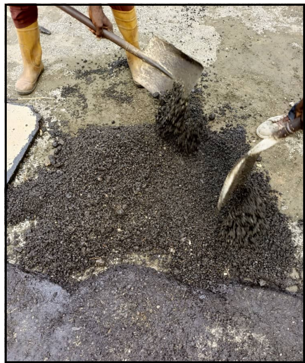
Fig. 19: The laid part and the mixture being done with shovels.
