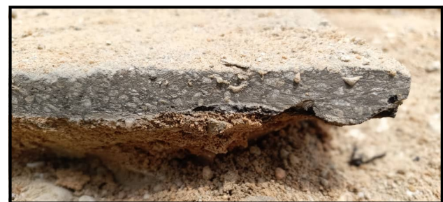
Fig. 16: The groove made under the asphalt.
