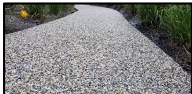
Fig. 11: Epoxy flooring with stone pebbles
