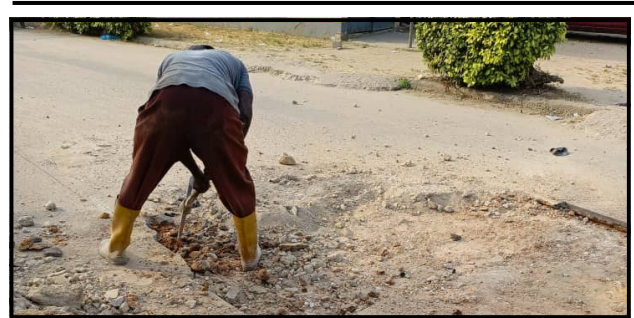
Fig. 14: The cut pothole being excavated..
