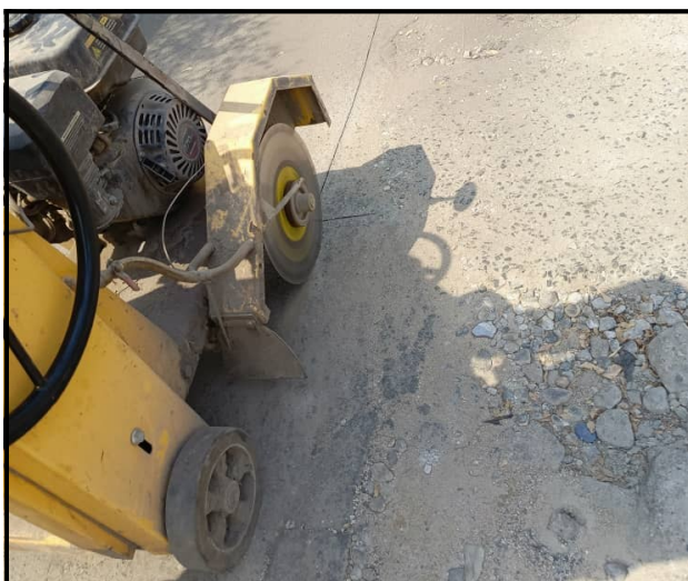
Fig. 13: Details showing the road being cut in straight lines.
