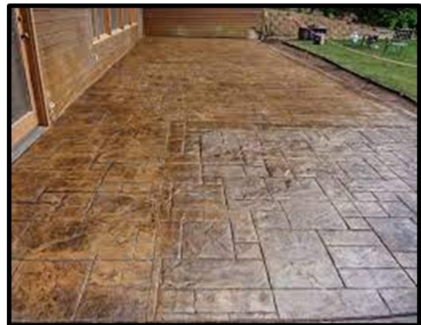
Fig. 10: Outdoor patio epoxy flooring. Source: https://www.cnycreativecoatings.com/residential/outdoor-patio
