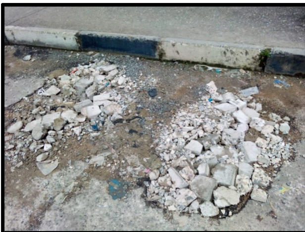
Figs. 1 and 2: Potholes filled with rubbles and sand at the entrance of University of Cross River State, Calabar. Note how the rubbles are loose and have gradually given way. Source: Authors, 2023.
