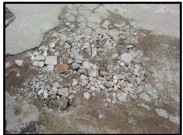
Figs. 1 and 2: Potholes filled with rubbles and sand at the entrance of University of Cross River State, Calabar. Note how the rubbles are loose and have gradually given way. Source: Authors, 2023.
